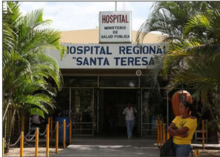
Hospital Regional Santa Teresa
