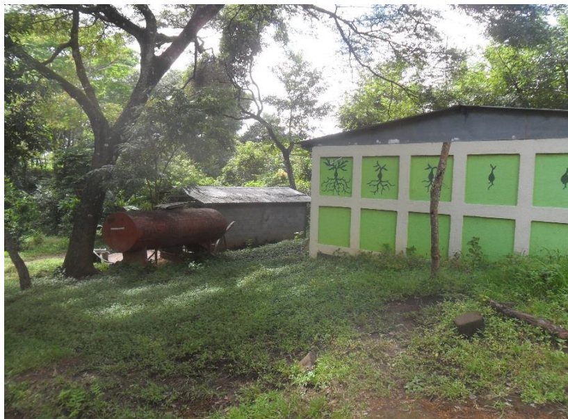
Entrada principal RAEME 3
