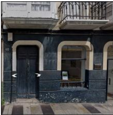
Frente a fachada Principal
