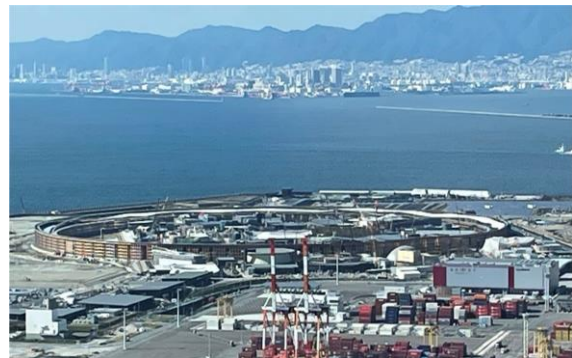
2025 Osaka Kansai Expo construction site view
