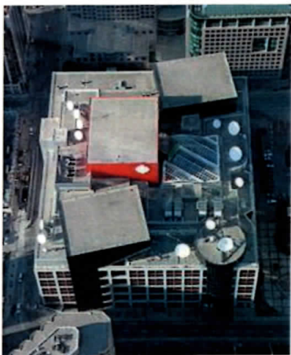
Ilustración 30 Canadian Broadcasting Centre, Canada - Philip Johnson
