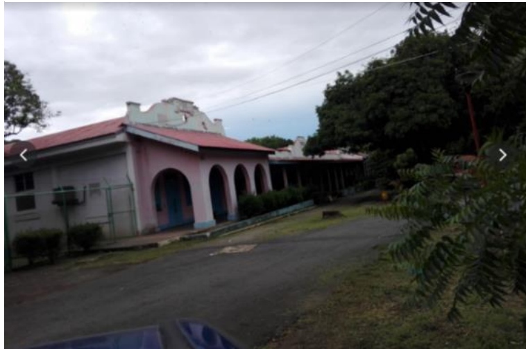
Fachada Hospital Psico Social Managua
