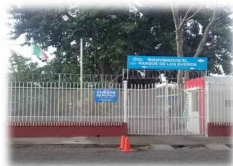
Foto 9. Entrada principal de Kingdom School.
